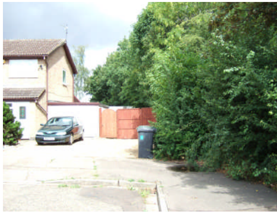
Fig 11: Trees encroaching towards a residential property.
